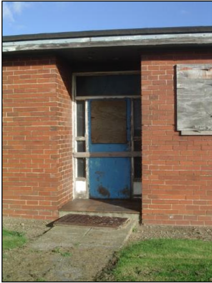
Photo 25: Building 2 front view
