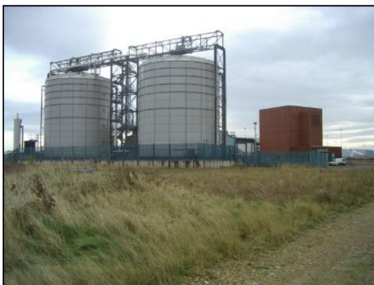
Photo 54: Sludge holding tanks
