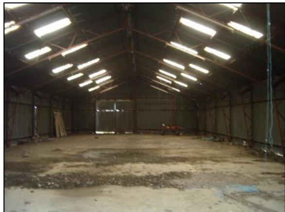
Photo 22: Building 2 internal view
