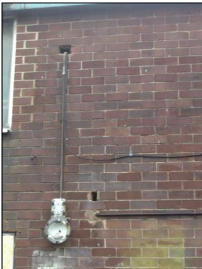
Photo 38: Annex external wall
