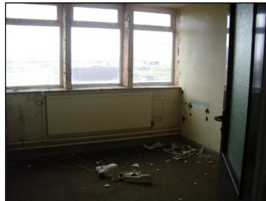
Photo 47: Building 9 first floor
