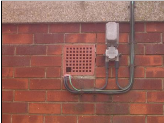
Photo 32: View of cut section airbrick
