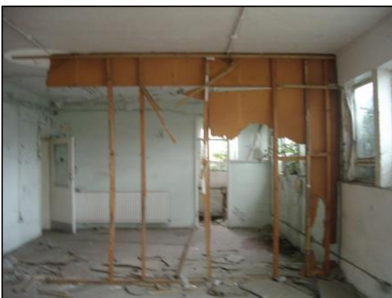
Photo 42: Internal view of building
