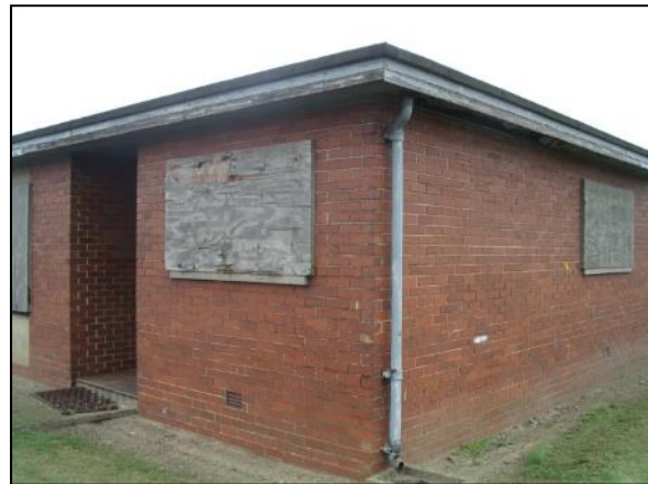
Photo 24: Building 2 close-up view
