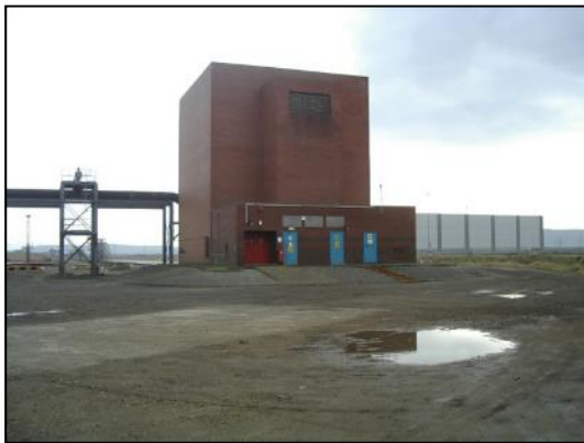
Photo 56: No.2 tunnel head house
