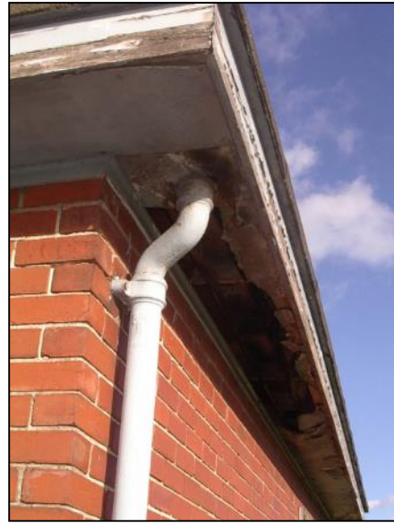
Photo 26: Decaying soffit-board
