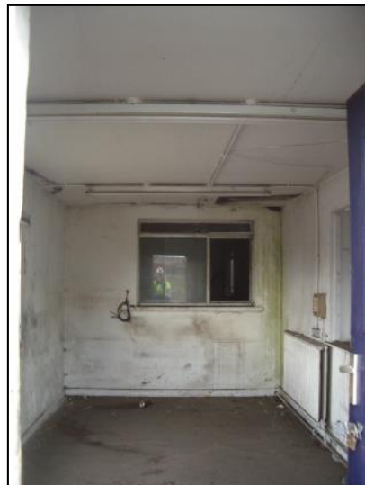
Photo 39: Annex internal view
